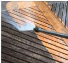
Routine maintenance needed to keep the original Teak color
